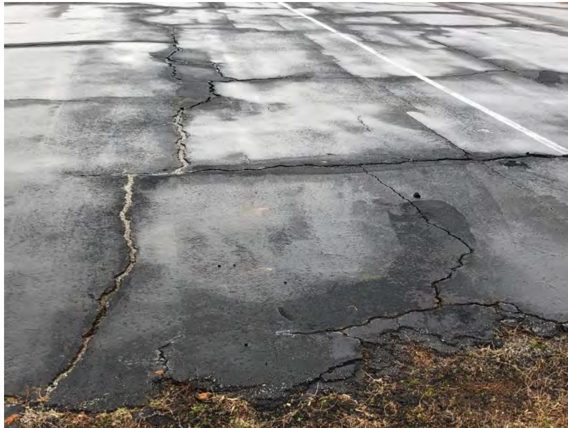
Cracking pavement at the R/C runway
